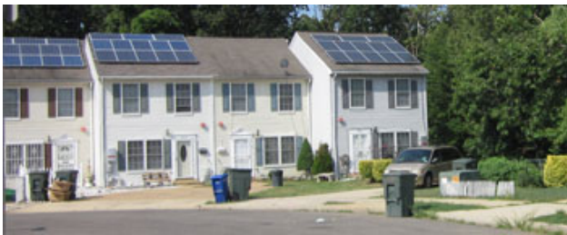
Fig. 5: Solar installations in Ward 8
