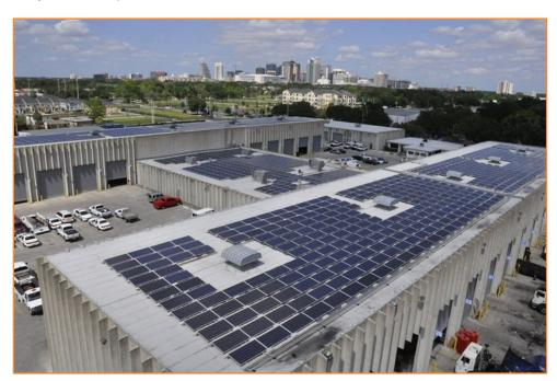
**Figure 3.** City of Orlando's Fleet and Facilities Compound with 420 kW Solar PV Array (Installed in 2013, Courtesy of the City of Orlando)
