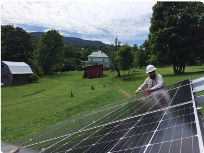
Installer puts panels into place on Rafe Pomerance's West Virginia farm.
